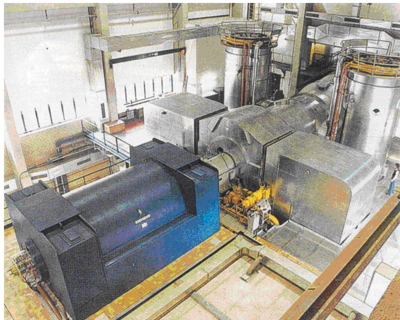
6 Leopoldau peak power plant, Vienna, Austria Erected by Siemens / KWU using AEG Static frequency converters Generator power: base load 85.0 MW peak load 93.5 MW
