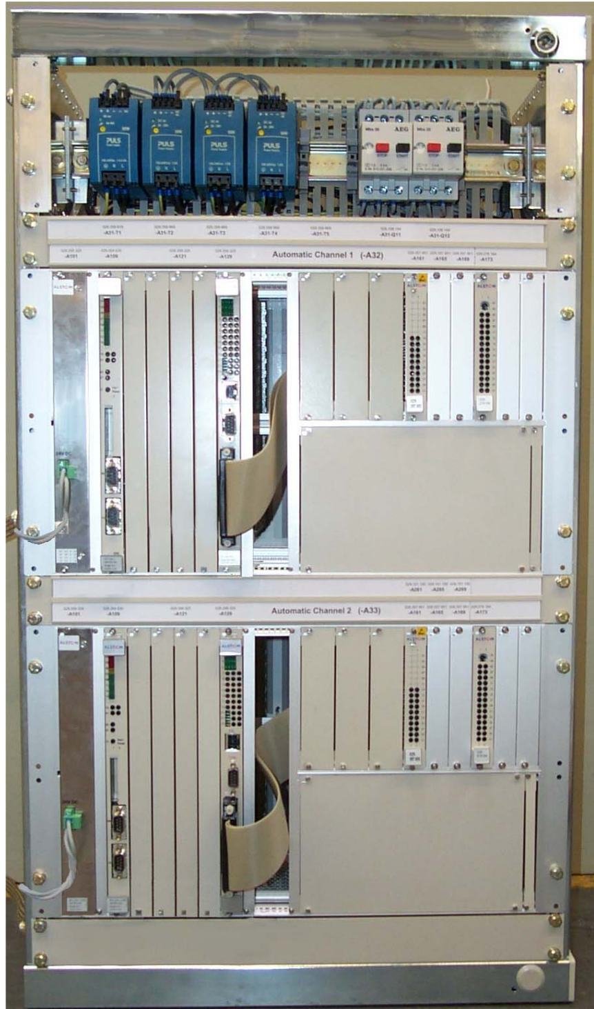
8 Hinged frame with plug-in cards for static frequency converter and excitation control. Two automatic control channels.
